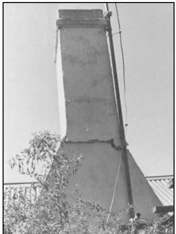
Earthquake damaged chimney, farmhouse near Robertson NSW (photo from Dayeh, 1976).
