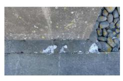
Figure 2. Concrete spalling at base of chimney, (looking downward)
