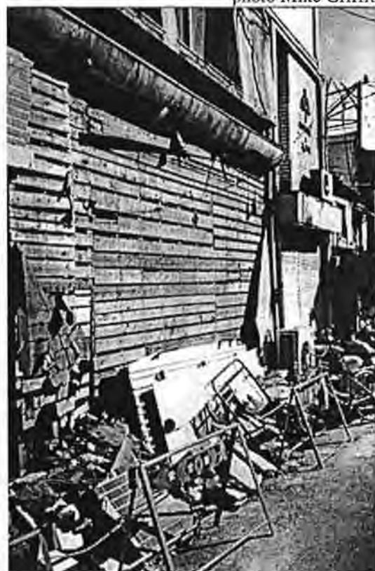
Fig 2 Cladding failure reducing lateral stiffness
