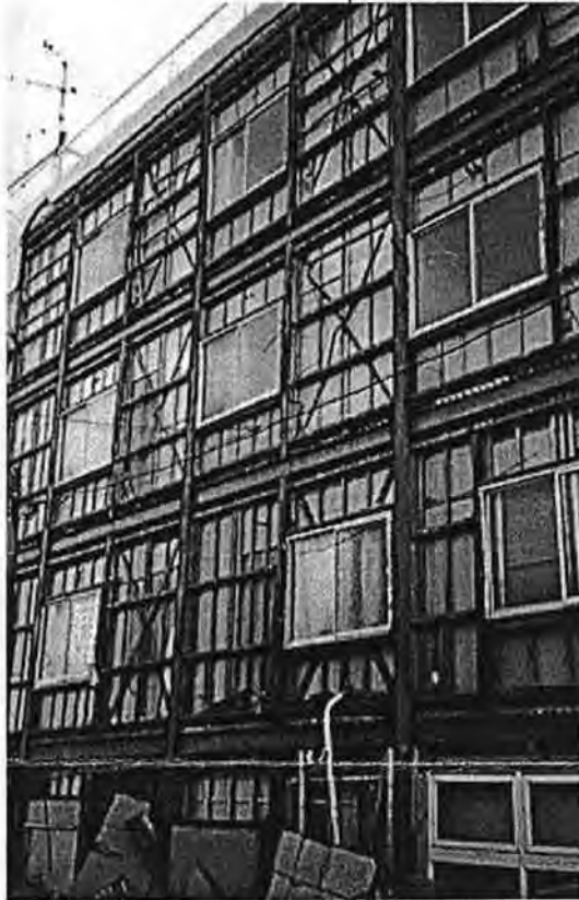
Fig 7 cross-braced steel frame with failed cladding
