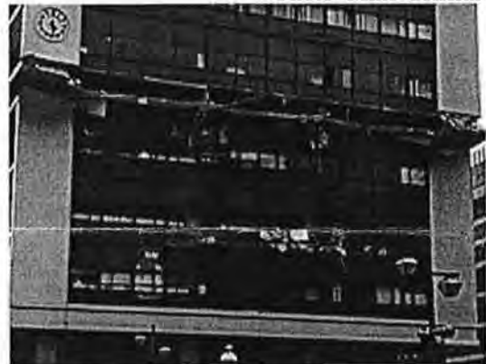
Fig 9 Collapsed upper storey of old Kobe City Hall building
