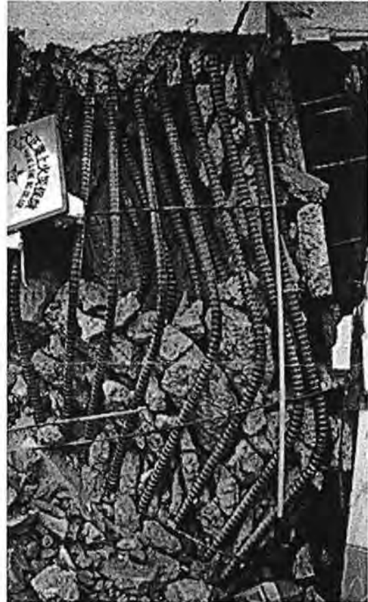
Fig 8 Large tie spacing led to many failures
