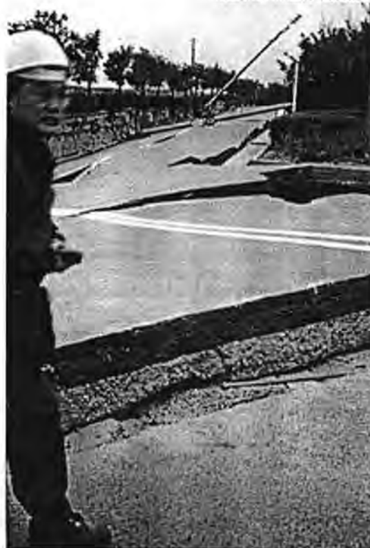
Fig 3 Lateral spreading - Rokko Is in port area
