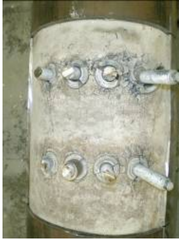
Figure 8 Concrete in circular column
