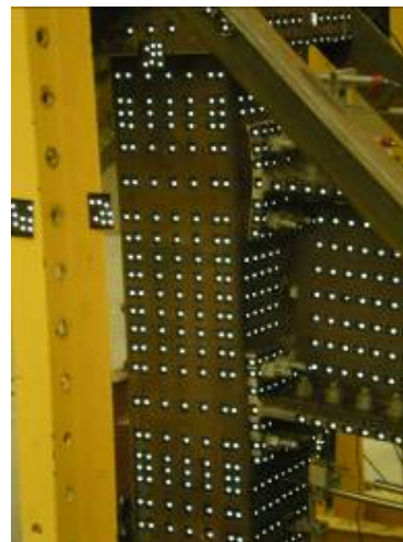
Figure 7 Failure of specimen 2
