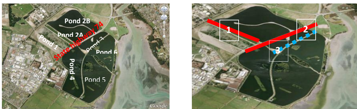
Figure 1: Christchurch wastewater treatment plant ponds location and damage (Google map)
