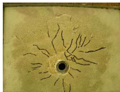
Figure 10 Concrete in specimen A_M20_N2
