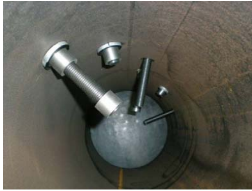
Figure 3 Blind bolts in the CHS
