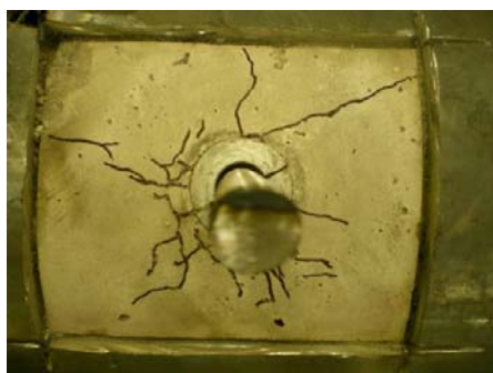
Figure 9 Concrete in specimen T6_D20_N2
