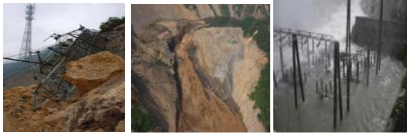
(a) electric-pole tilt down (b) reservoirs filled by landslides (c) inundated power equipments Fig.4. Power supply system typical earthquake damage
