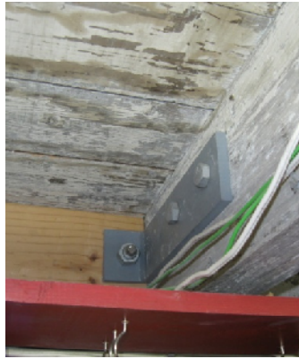
(b) joist-wall connection
