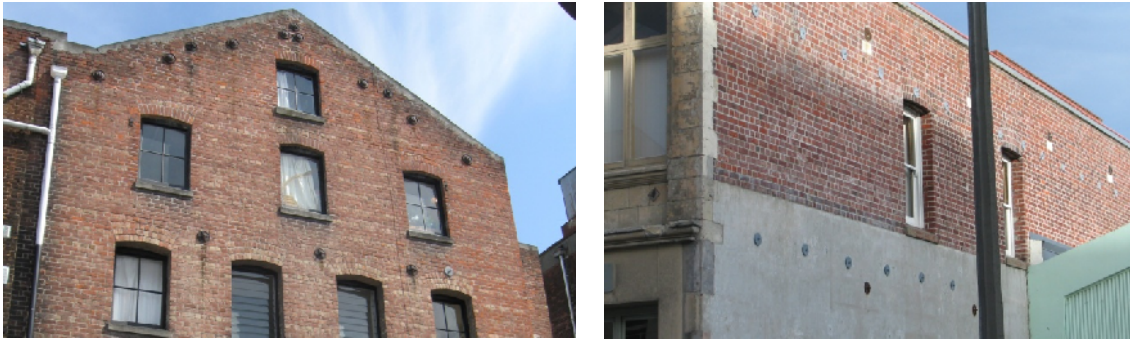
Figure 16. Successful wall-floor and wall-roof diaphragm anchorages.
