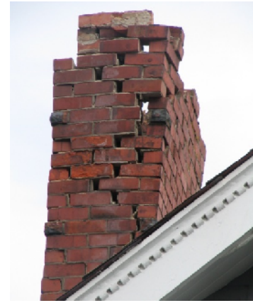
(b) Unstable damaged chimney
