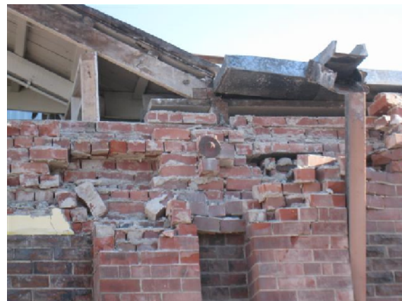
(b) Wall anchor still intact
