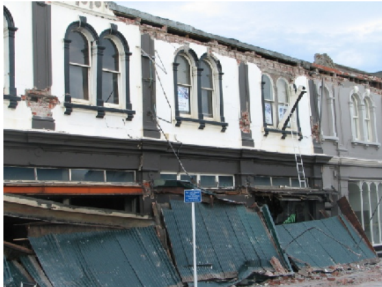
(a) Multiple front wall parapet failures
