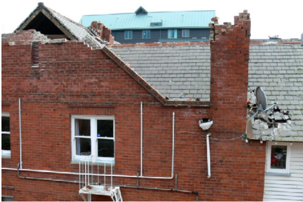
(a) Two damaged chimneys and gable wall.
