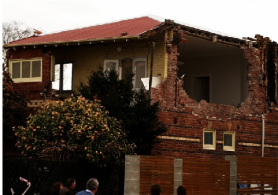
Figure 10. Examples of out-of-plane failures in cavity walls.
