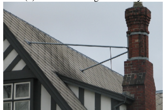
(d) Braced chimney performed well
