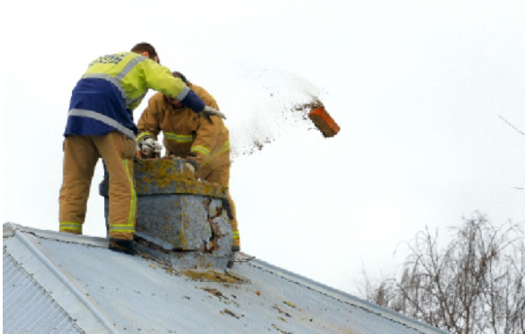
(c) Emergency services remove chimney.
