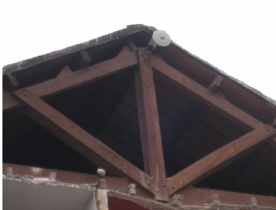
(a) Gable wall failure despite anchor
