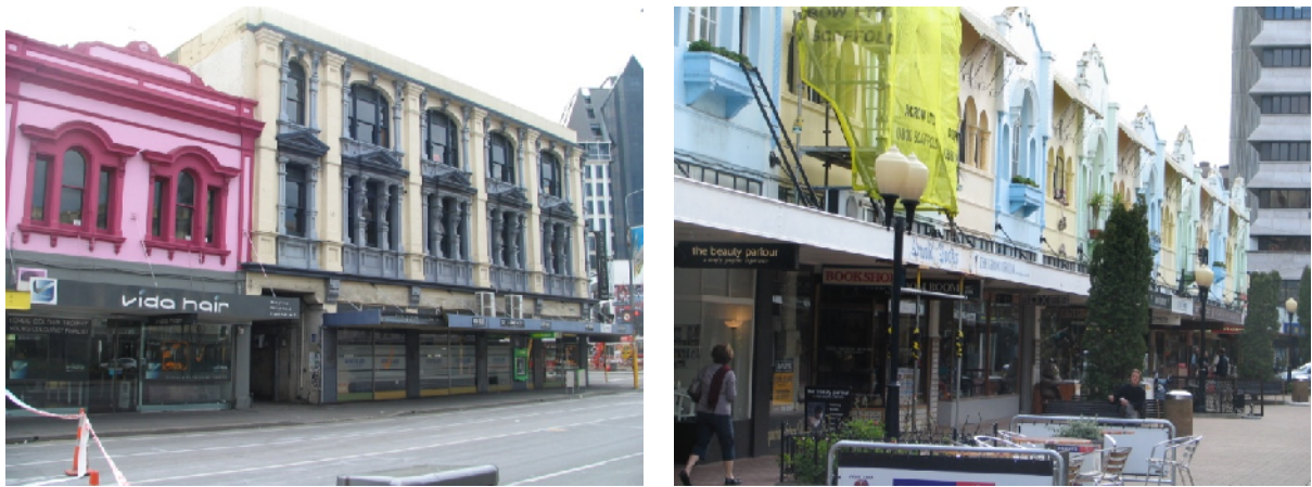
Figure 4. Typical 2- and 3-storey URM buildings in Christchurch.
