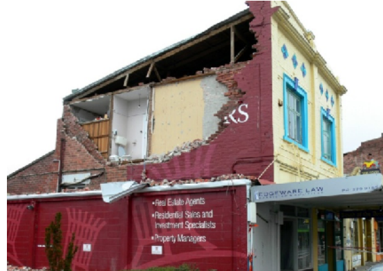
Figure 10. Examples of out-of-plane failures in cavity walls.
