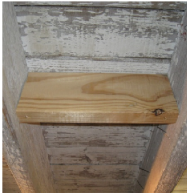
(a) blocking of joists
