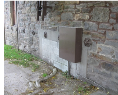
(c) diaphragm anchors – external view
