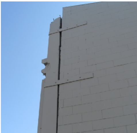
Figure 21 – Examples of corner ties
