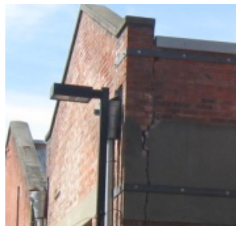
Figure 21 – Examples of corner ties
