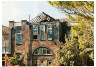
with a brick or stone chimney. The Workers Club was the only building that suffered partial collapse but many houses lost chimneys and some moved off their timber piles and suffered puncture failure. The latter type of damage was often not observable from a brief streetside inspection, the house still looked level, the chimney lying in the backyard. The only sign of a problem was the disconnect between the front steps and entrance.
