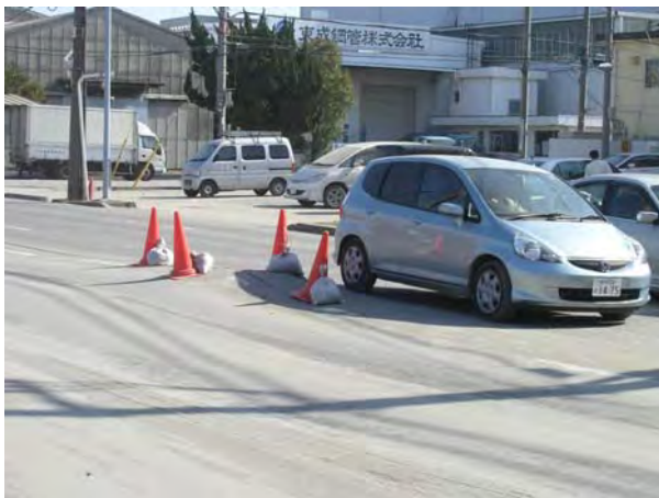
Fig. 22 Satisfactory performance of major road in Urayasu
