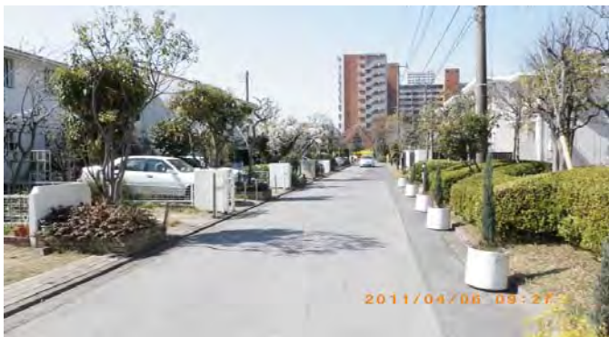
Fig. 26 Successful soil improvement by gravel drains against liquefaction
