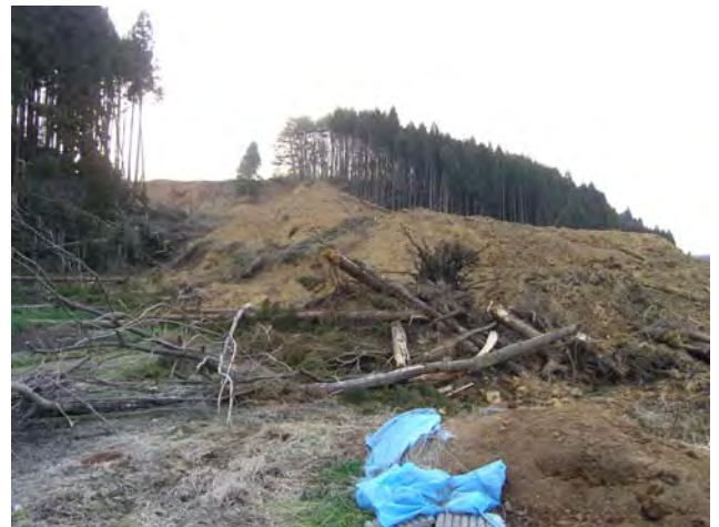
Fig. 8 Failure of natural slope in Shirakawa City
