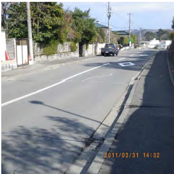
Fig. 11 Relatively intact shape of residential development in cut part
