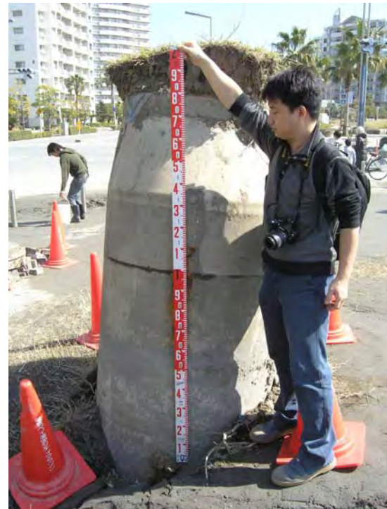
Fig. 19 2-meter floating of manhole
