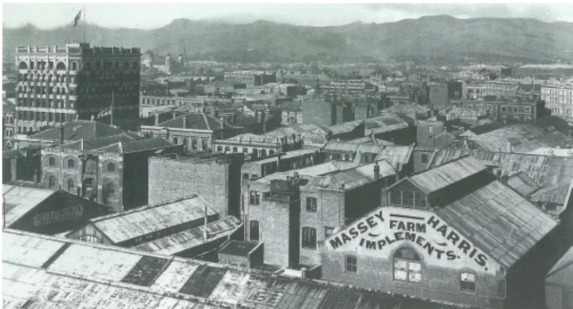
Figure 3 New Zealand Express Company building, Christchurch's first 'skyscraper', photo circa 1910 (Brittenden Collection, 1910)
