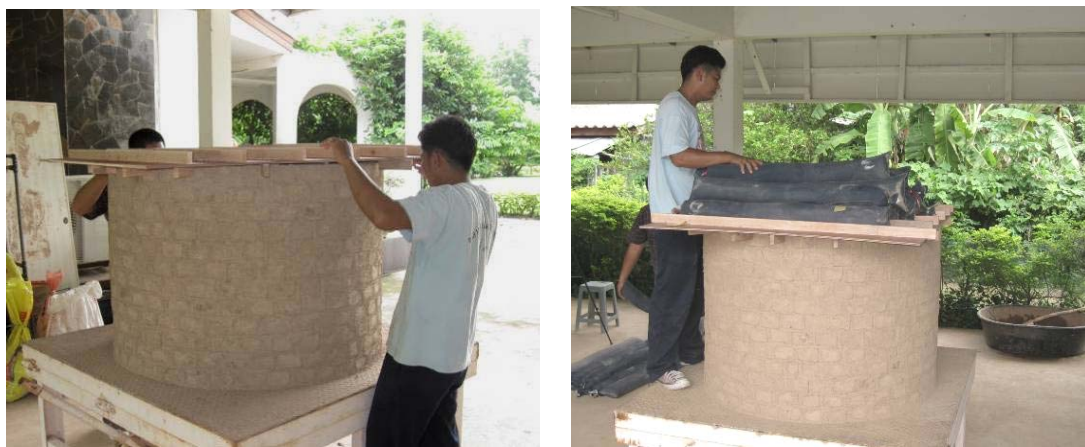
Figure 2: Roof and sand bags installation.
