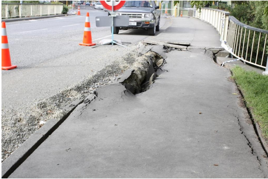
Figure 15. Subsidence of fill behind the abutment
