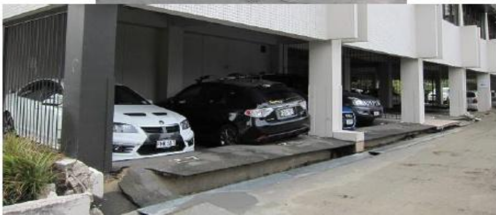
Figure 16. Tilting of building caused by liquefaction (Photo by Wen Kam)
