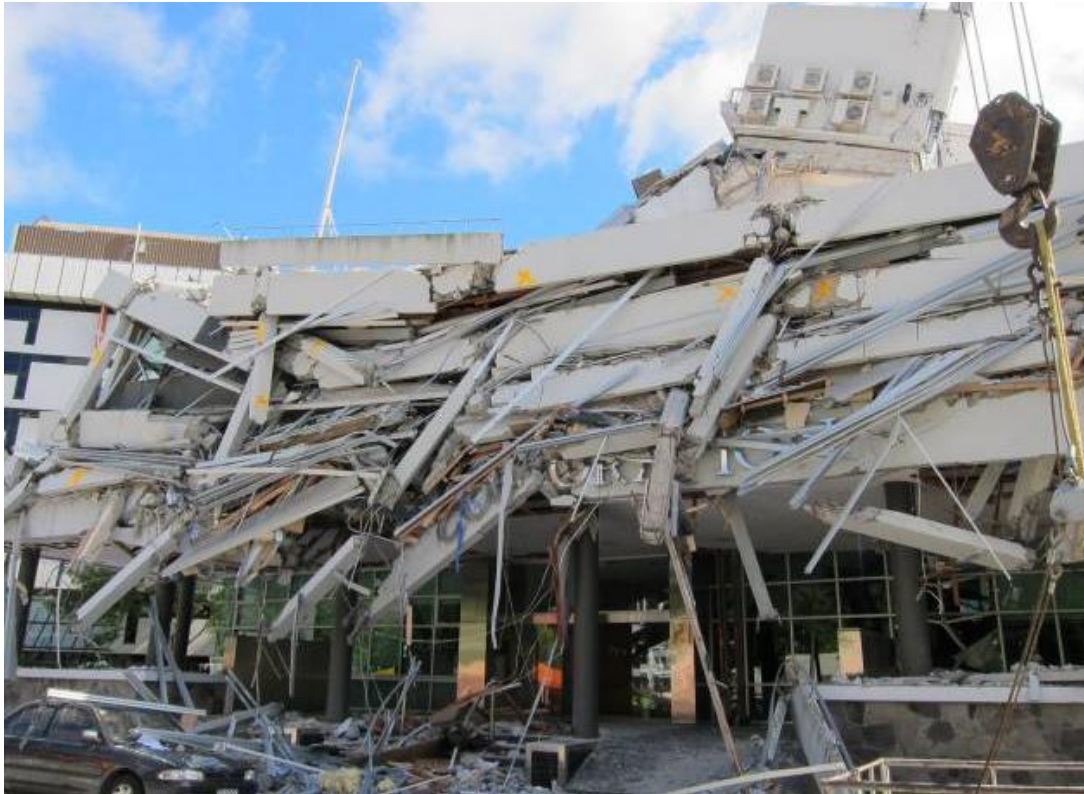
Figure 7. Pyne Gould collapse from the southern side
