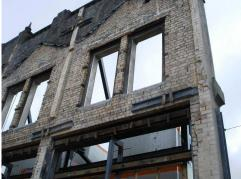
Figure 1: A section of a three-storey demolished building; stepped exterior walls and two-leaf uniformthickness interior walls are visible
