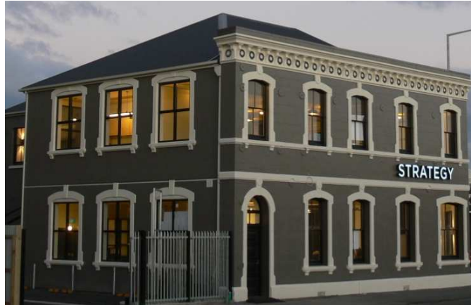
Figure 7 - Successfully retrofitted Christchurch URM building (May 2011)
