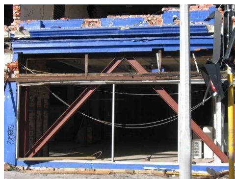
b) URM building with visible retrofit
