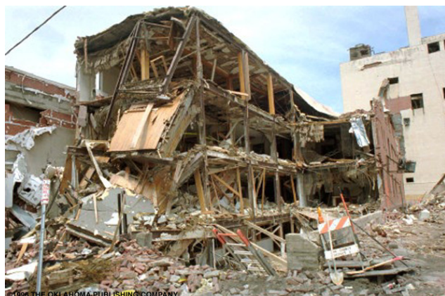
Figure 3: Disproportionate collapse — Oklahoma 1995
