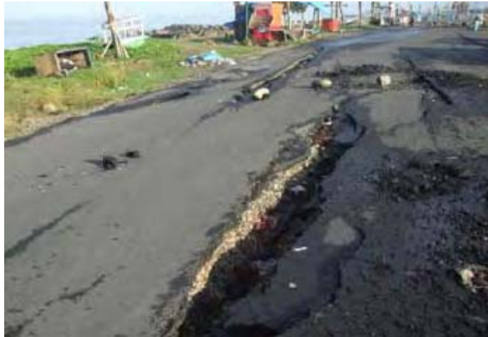
Figure 6 – Ocean boulevard liquefaction. Note low elevation affording minimal tsunami protection
