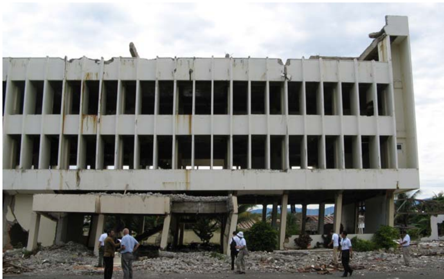
Figure 4 – Provincial Public Works Office, Padang Evidence of soil liquefaction at this site
