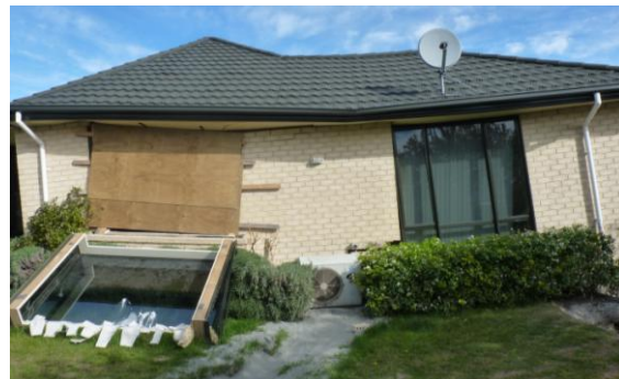
Figure 2 Liquefaction damage
